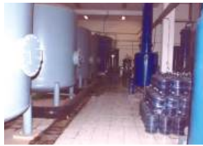
EcoBeam XL Installation on a Jet PackClarifier and Automatic Valvless Gravity Filtration System with Capacity of 60m 3 per hour
