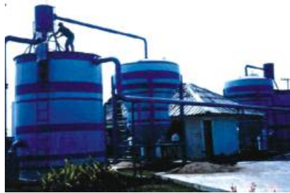
EcoBeam XL Installation on a Jet PackClarifier and Automatic Valvless Gravity Filtration System with Capacity of 60m 3 per hour
