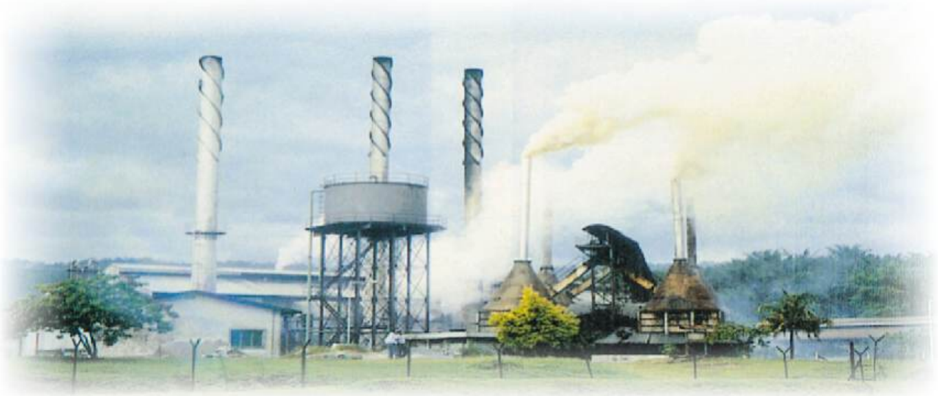
An Oil Mill with EcoBeam XL Treatment System
